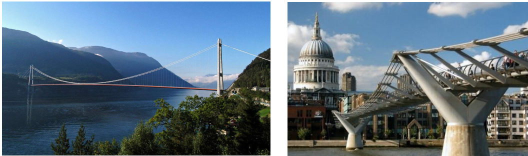
Figure 1.1. Left: Hardanger Bridge, Norway. 1 Right: London Millennium Bridge, UK. 2
