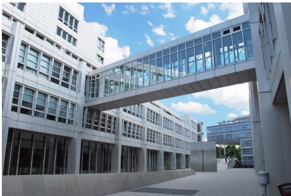
Figure 18 – OEB Munich, complexe PschorrHöfe
