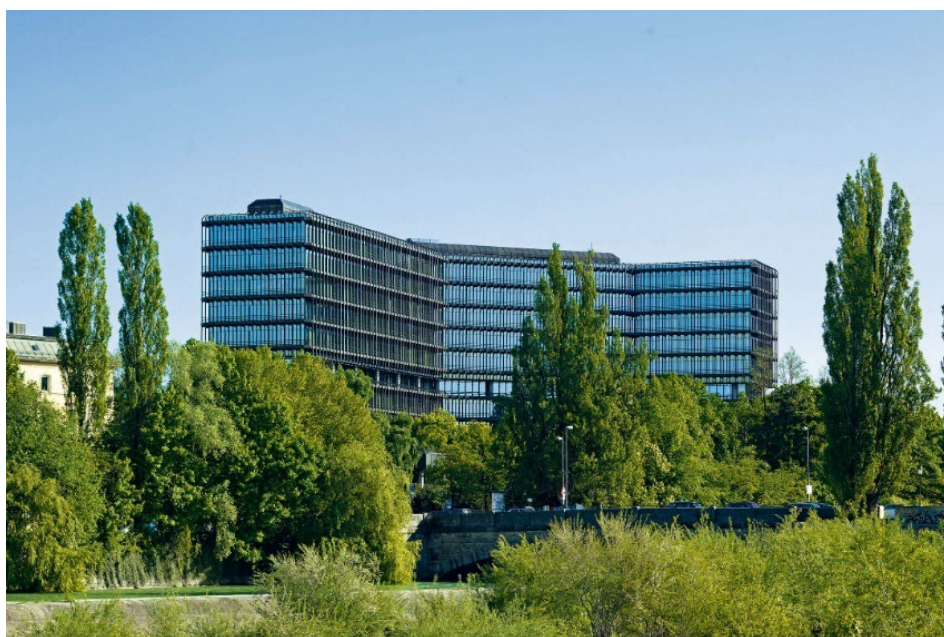
Figure 17 – OEB Munich, bâtiment Isar
