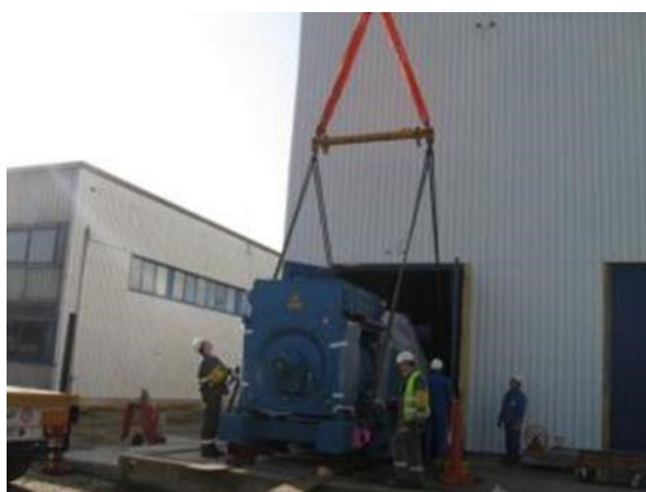
Figure 24: Installation of new safety diesel generators in the DGG of units Doel 1 & 2
