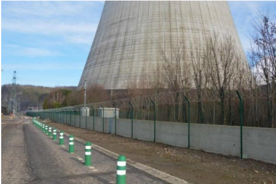
Figure 17: New peripheral protection of the site of Tihange
