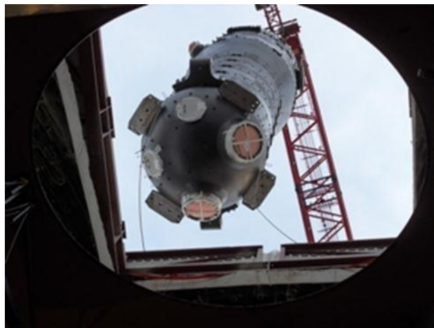
Figure 23: SG Replacement at Doel 1
