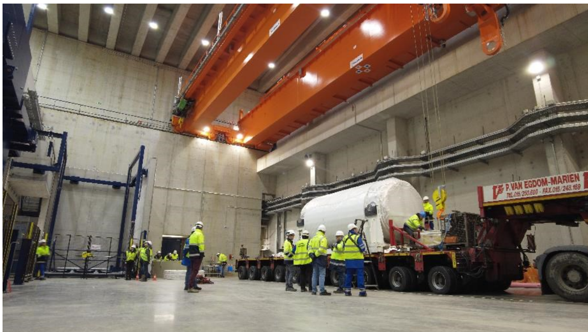
Figure 32: Arrival of the first spent fuel cask in the Intermediate Storage Building for Spent Fuel of Tihange
