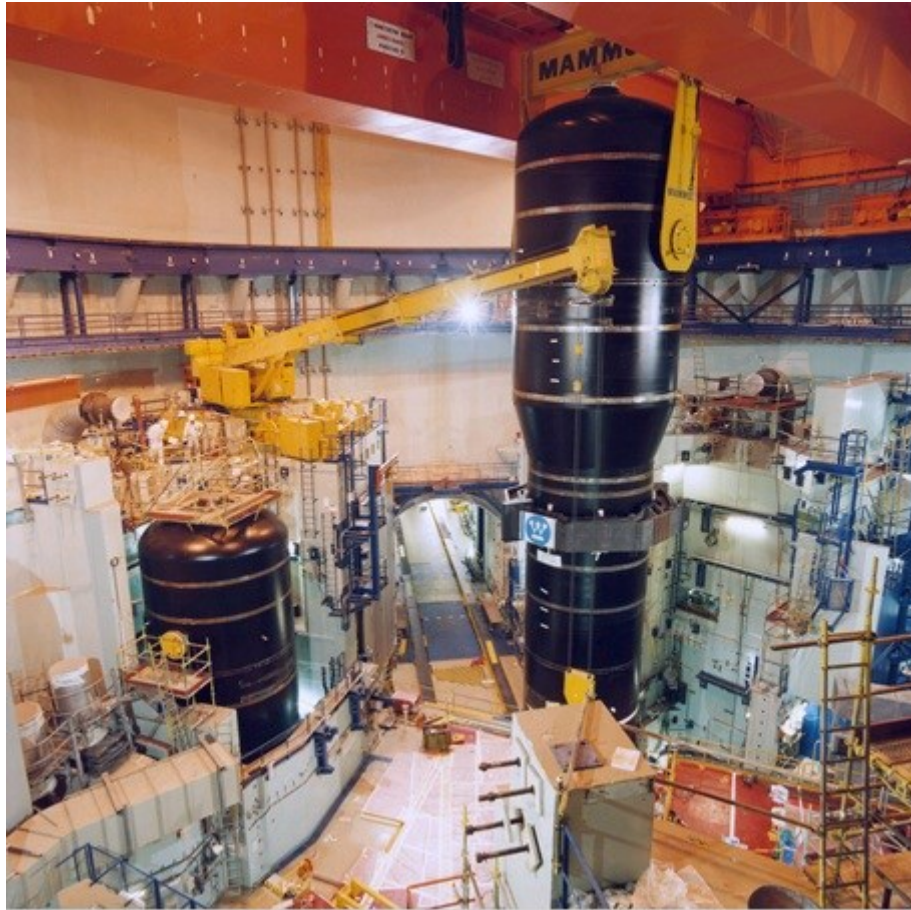
Figure 28: Replacement of SGs of Tihange 3
